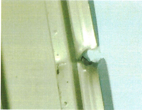
TYP. PANEL TEAR AT SCREW LEG
